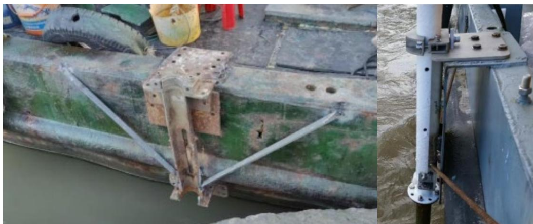
Figure 2-5 Support soudé et monté
